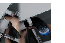
5. Secure the main unit to the ceiling joists, then connect the ductwork and power supply.
