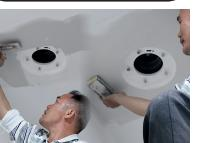
7. A carpenter applies putty with a brush to finish ceiling repair.
